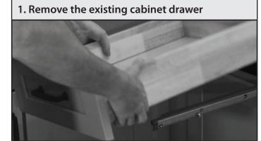
Remove the existing drawer, keeping the drawer front and any decorative hardware to reuse in Step 6.
