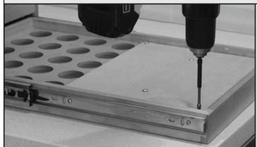
Slide the upper shelf rearward and turn upside down. Position one or both support boards as shown, and secure with the  $#8 \times 1/2''$  pan head screws provided.
