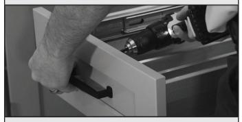
Install the drawer front and decorative hardware onto the double drawer unit.
