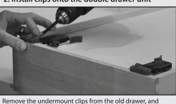
Remove the undermount clips from the old drawer, and install them onto the double coffee drawer bottom. New clips are sold separately, if needed.
