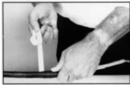
FIGURE 13 – APPLYING LOCK-TAPE SEALANT
