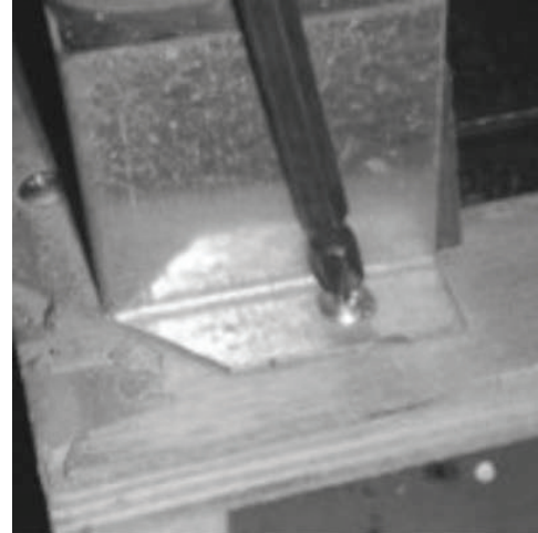
Image 2: Removing bracket from cabinet
