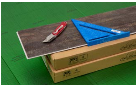
Cutting boards using Score and Snap technique
