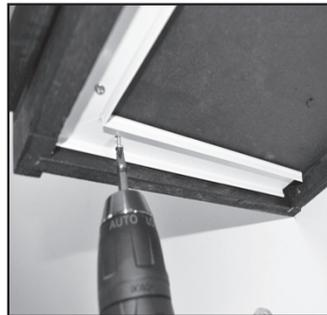
5. Snap lens onto fixture. Position fixture in center of cabinet and snap into WireWay Base.
