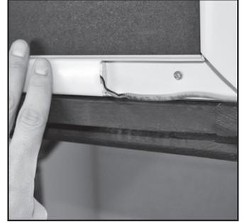
2. Cut WireWay Base to fit full length of cabinet face. Deburr cut edges. Using screws provided, secure Base to bottom of cabinet every 12". (When wiring between adjacent cabinets, drill 1/4" hole through end panels.)
