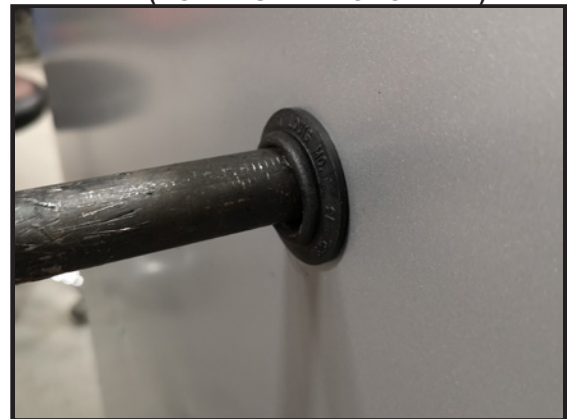
FIGURE 28 - FURNACE GAS PIPE CONNECTIONS (NOTE RUBBER GROMMET)
