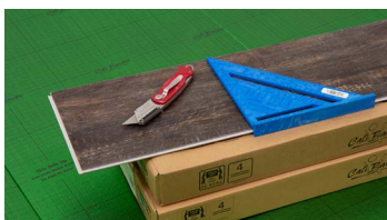
Cutting boards using Score and Snap technique
