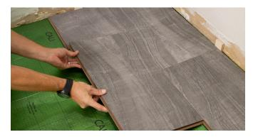
2. Install second plank by angling long side of the plank and gently sliding until the butt end seams are in contact, and then gently tapping all seams into place. After installation is complete remove all 1/2" spacers and insert 3/8" compressible PE foam backer rod. Seal expansion space with 100% flexible silicon sealant. DO NOT use acrylic-based sealant.
