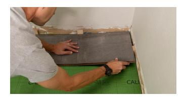
4. When you reach the wall, cut the tile no less than 6" to fit while maintaining the 1/2" expansion gap.
