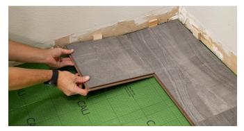
1. Start new rows with pieces trimmed from previous rows that are at least 12" in length and ensure a minimum end joint offset of at least 1/3 the length of the plank. At a slight angle, insert tongue into the groove of the plank from the previous row until the laminate edges meet. Angle down until the joints lock.
