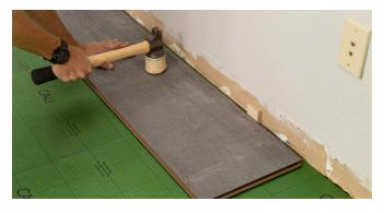
3. Ensure that the planks remain aligned and the joints stay securely closed throughout the installation process. Continue in this manner until reaching the final board in the first row.
