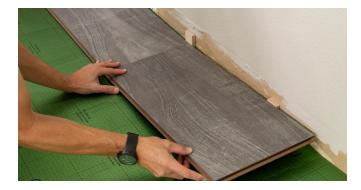
Install the second piece by aligning the butt end with the end of the first piece at an angle. Gently push the second piece down until the tongue and groove lock together to secure the end joint. The planks should lay flat.
