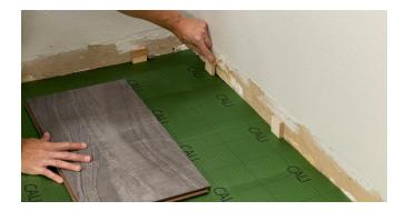
Starting from the left, place the first plank with the tongue side facing the wall. Throughout the entire installation process, remember to check that your spacers are maintaining the 1/2" expansion space along room perimeter or next to any fixed objects.
