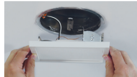
Friction clips for recessed housings
