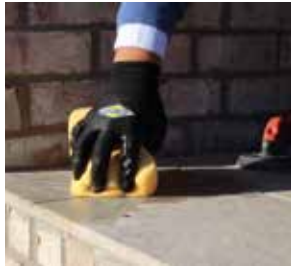
PIC 2. Remove excess grout with clean water.
