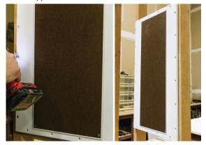
Once the board has been properly leveled, fasten the PBF board to the vertical and horizontal studs.
