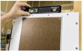
After this has been done, ensure that the board is level before fully securing it to the wall studs.
