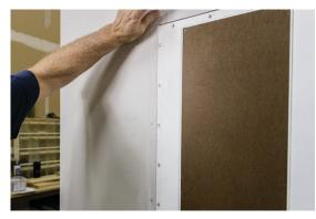
Now, cover the seams around the board with mesh tape, and begin the mudding process.
