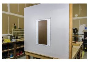
Cay the frame panel of sheet rock over the PBF board and fasten the frame to study of the wall.
