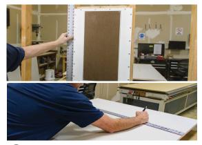
Measure the PBF board and make an outline of the board on a new panel of sheet rock.
