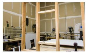
Before installing the PBF pre-construction board, we recommend securing two horizontal studs, at PBF board height, between the vertical studs of the chosen installation location to add additional support.
