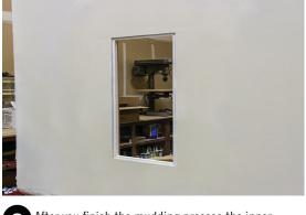
After you finish the mudding process, the inner plug can now be removed and sanding can be performed to remove any unwanted surface features.
