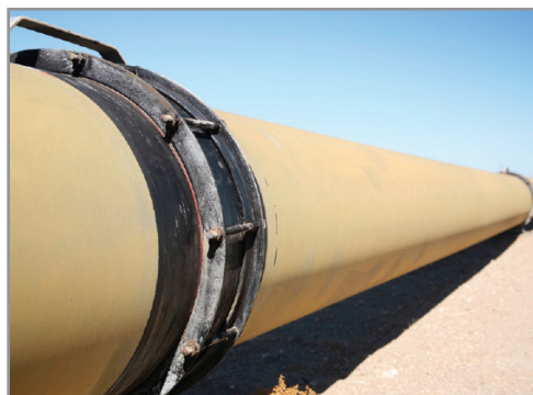
Tape application on oil pipeline.
