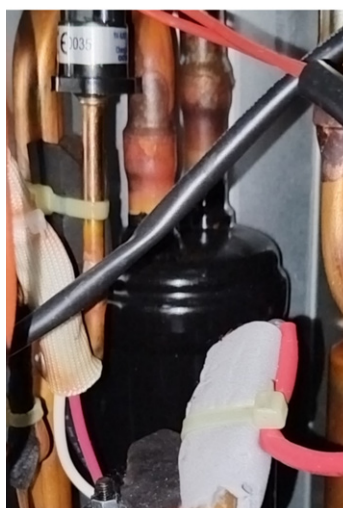
Gas-Liquid Separator
