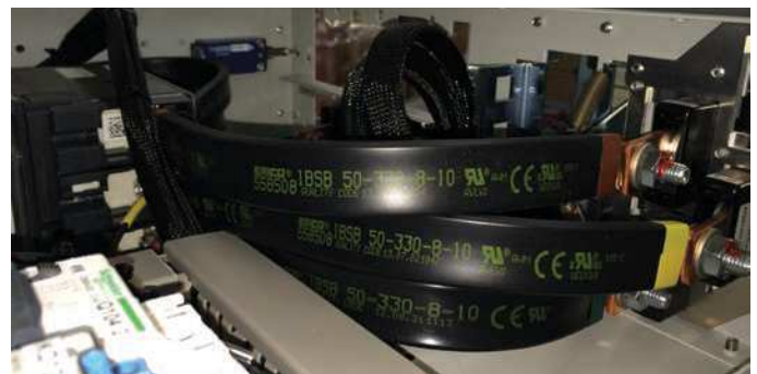
Figure 10 – nVent ERIFLEX IBSB used in tight spaces
