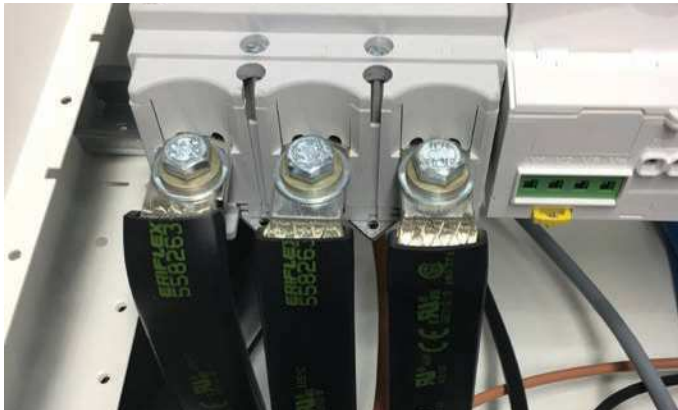
Figure 7 – Close-up view of the nVent ERIFLEX IBSB Advanced termination as installed
