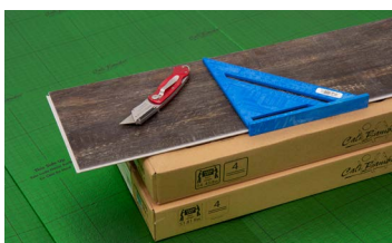
Cutting boards using Score and Snap technique
