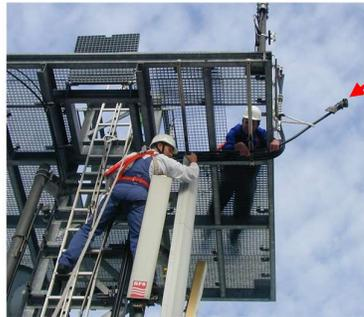
**Protective measures: temporary fixation of the cable**
