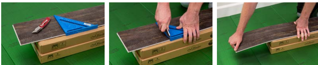
Cutting boards using Score and Snap technique
