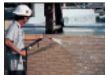
Panel is cleaned to remove concrete leakage.
