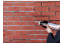
Mortar is installed into the brick joints with a grout bag or with mortar dispensing gun.
