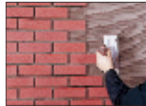
Mortar is applied with a 1/4" notched trowel.
