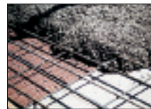
After steel reinforcing is in place, concrete is poured over the assembly.
