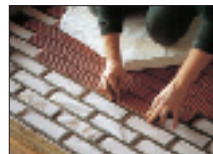
Brick are placed over retarder paper in gasket liner
