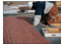
Assembly of Brick Snaps for Tilt-Up is fast at the rate of 2 to 3 square feet per minute, per man.
