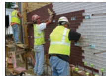
Thin brick is pressed into the pockets of the Rim Snap system face down.
