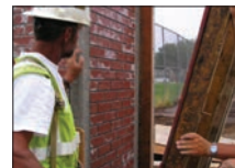
Forms are removed and the finished wall is power-washed to reveal a classic brick or stone finish in the structural concrete wall.
