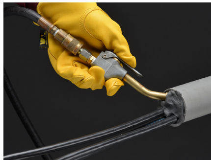
Blowing CableFree through conduits
