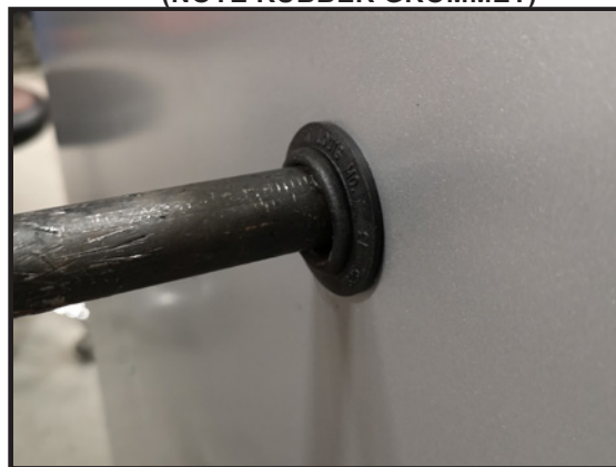
FIGURE 28 - FURNACE GAS PIPE CONNECTIONS (NOTE RUBBER GROMMET)
