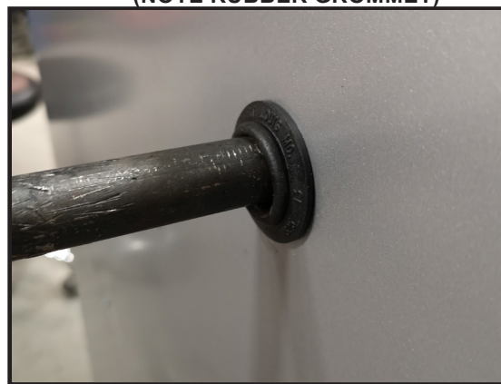
FIGURE 28 - FURNACE GAS PIPE CONNECTIONS (NOTE RUBBER GROMMET)
