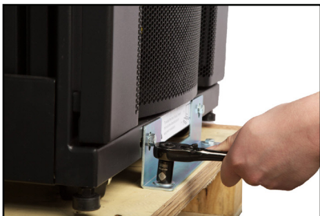
Removing the Bolts
