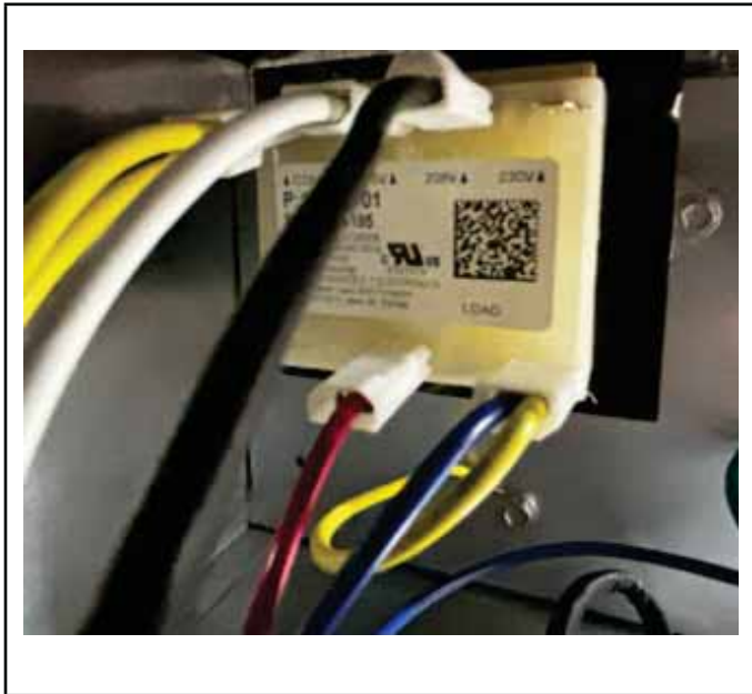
Figure 25. 230 TO 208 Voltage Conversion
