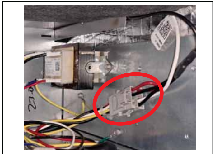
Figure 27. Converting Unit from 240VAC to 115VAC
