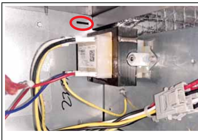
Figure 22. Notch for Control Panel Relocation
