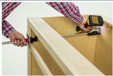
Attach slide bracket with screws using a drill or screwdriver.
