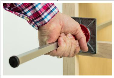
With your hand, grasp installation tool handle and place it in the bottom left corner of drawer opening. Be sure that the handle is flush and square against face frame.
