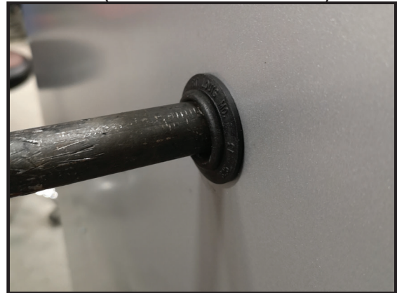
FIGURE 28 - FURNACE GAS PIPE CONNECTIONS (NOTE RUBBER GROMMET)
