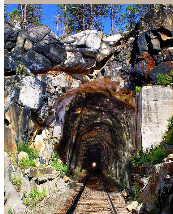
A view through Summit Tunnel from the west
