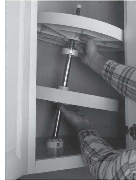
From the top slide one (1) Shelf Assembly, the other Shelf Support and then the other Shelf Assembly onto the Pole Assembly as shown. Slide bottom of Pole Assembly into the lower mounting support.
