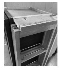
To ensure proper closing of the unit the rear of the filler may need to be adjusted. Extend the pullout so that the front is flush with the face frame or front of adjacent cabinet. If the filler front is not even from top to bottom, press down or pull up on the rear of the filler to make the filler front and face frame even. Install screws into rear mounting holes at this time. NOTE: Install remaining cabinetry, face frame, and/or door front (not provided).
