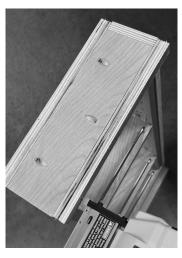
Install upper and lower scribe rails to the filler pullout using small finish nails or brads (not included). Upper and lower scribe rail is attached to the outside frame rail of the pullout as shown.
