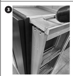
Mount pullout filler to adjacent cabinet installing screws into the frontmost holes on the top and bottom of filler's frame.
