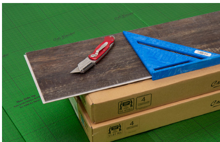
Cutting boards using Score and Snap technique
