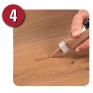
Cut tip to desired bead size and apply the filler evenly.
