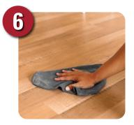
Wipe off excess with a damp rag. Do not allow excess filler to dry onto surrounding flooring.
