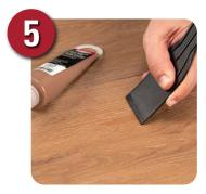
Use a putty knife to distribute into gaps, nicks and scratches.
