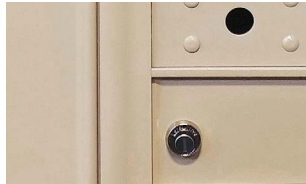
Interlocking, overlapping seams to prevent prying
