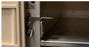
Easy release handle to open master gate
