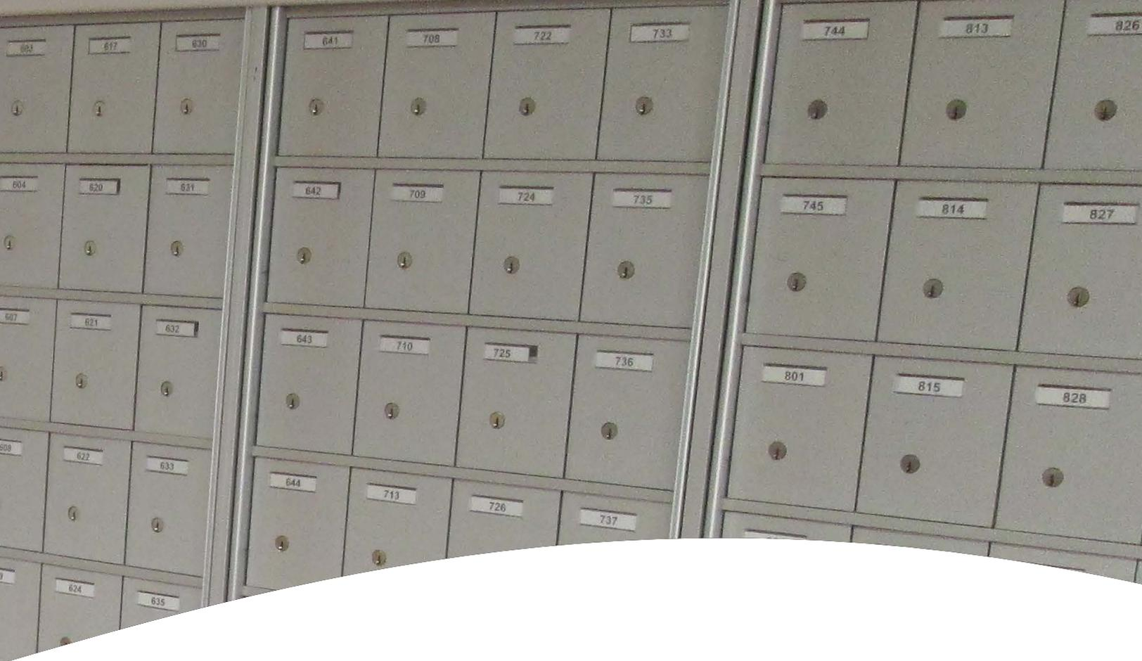
Vertical mailboxes come in five standard sizes and easily slip into the opening vacated by an older box; however, it is highly recommended that existing vertical mailboxes be upgraded to either a CBU or STD-4C to ensure proper security. As mail is loaded from the top of these vertical units, it makes them vulnerable to the weather so they should be used indoors only.
